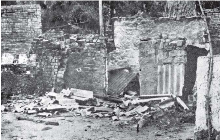
Rebuilt repeatedly—only to be shattered once more
