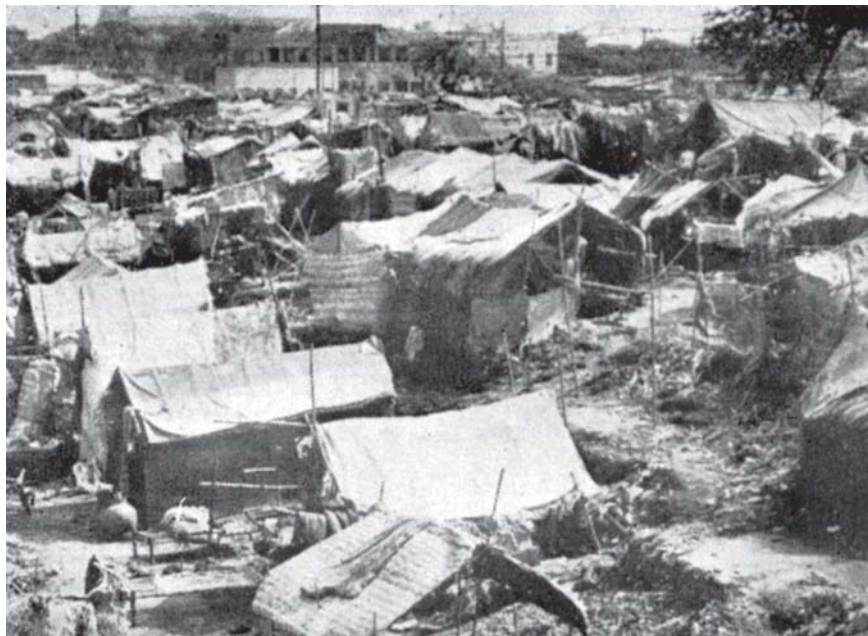
View of part of a Bombay slum
