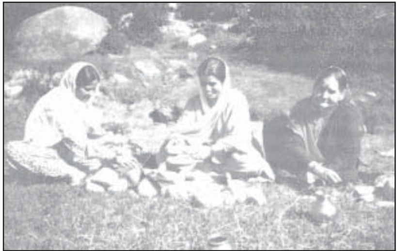
Kangra women : Building houses for Tulsi
